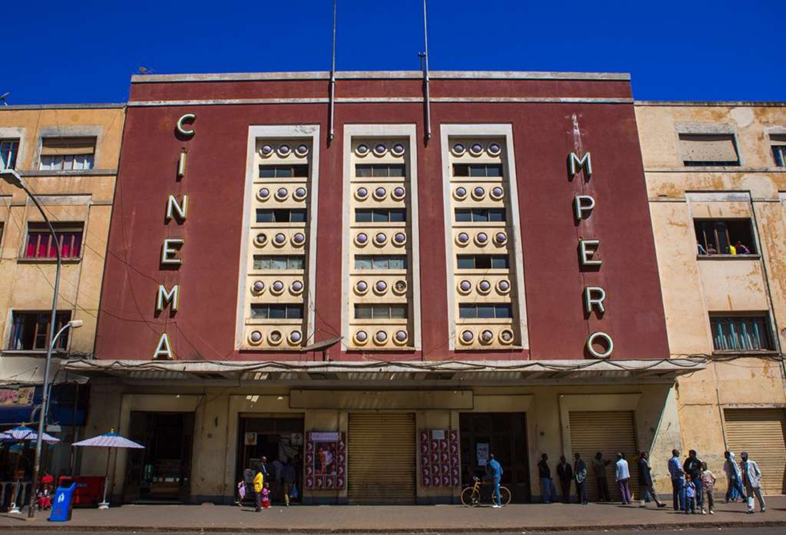
Cinema Impero on Liberation Avenue, built in 1938. The Cinema is made up of three massive windows with 45 porthole lamps. The auditorium can welcome 1800 people.
