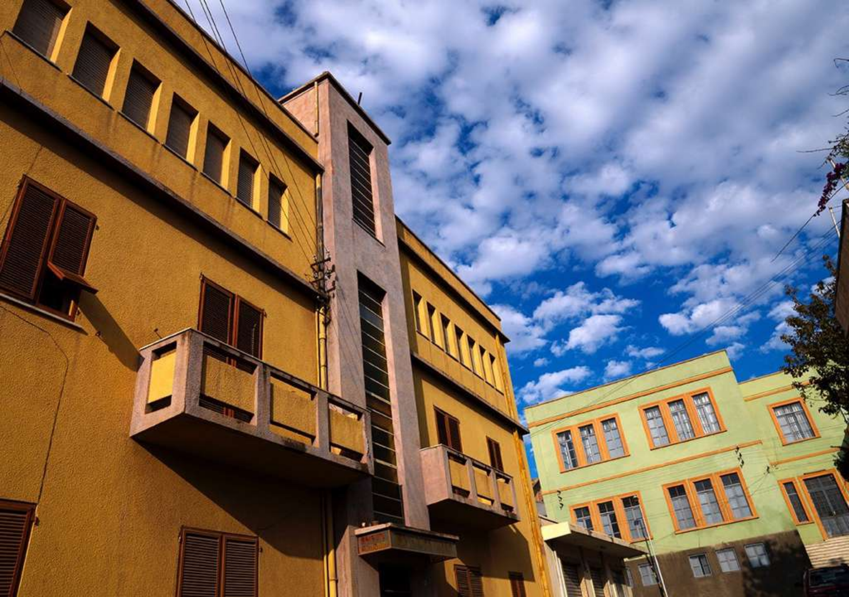
Former apartments build in the 40s, that became the « Bristol Pension » during the british administration.
