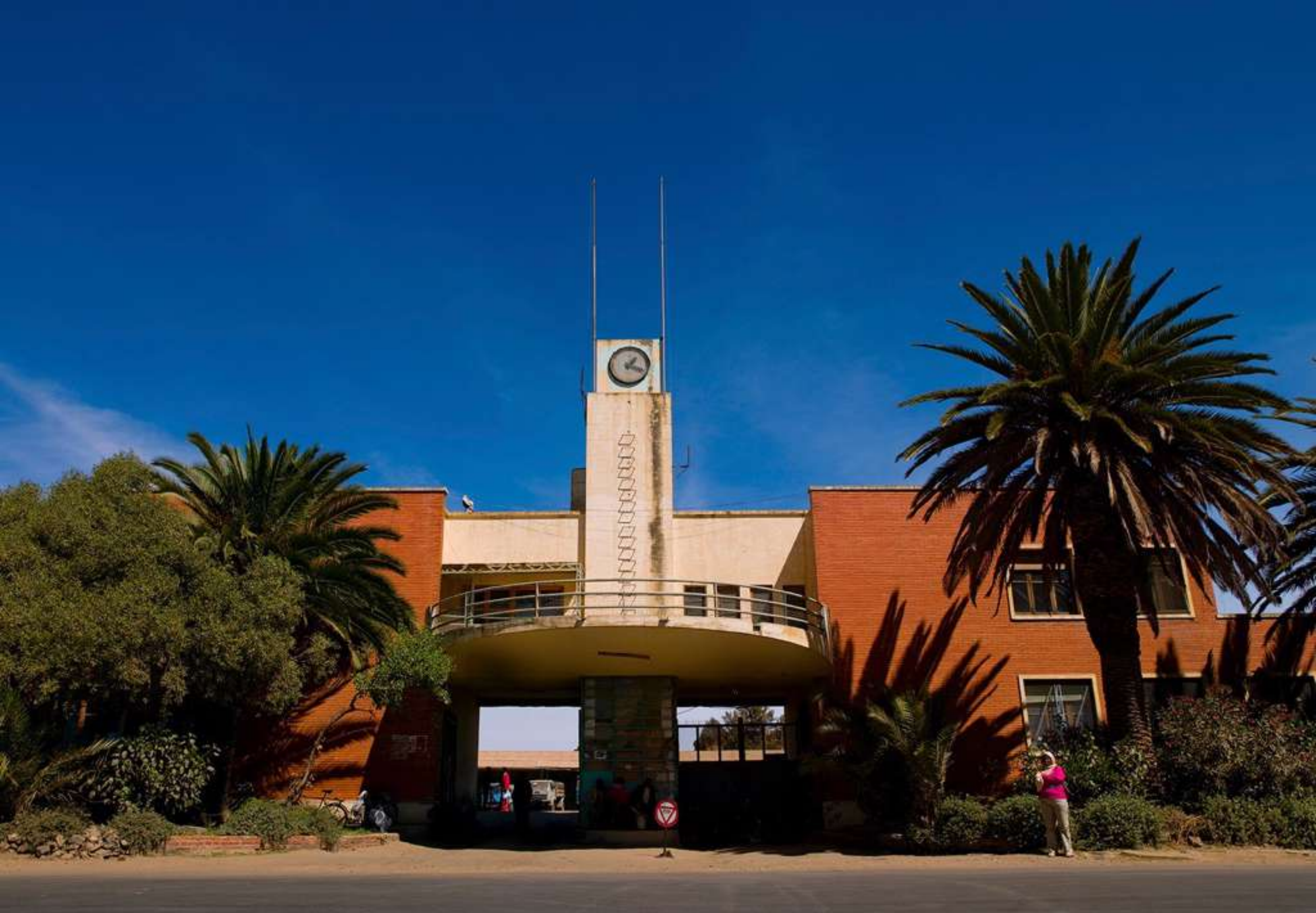
Former City Sanitation Modernist office turned into a garage on Massawa road. Lot of factories were also built in the city of Dekemare by italians.
