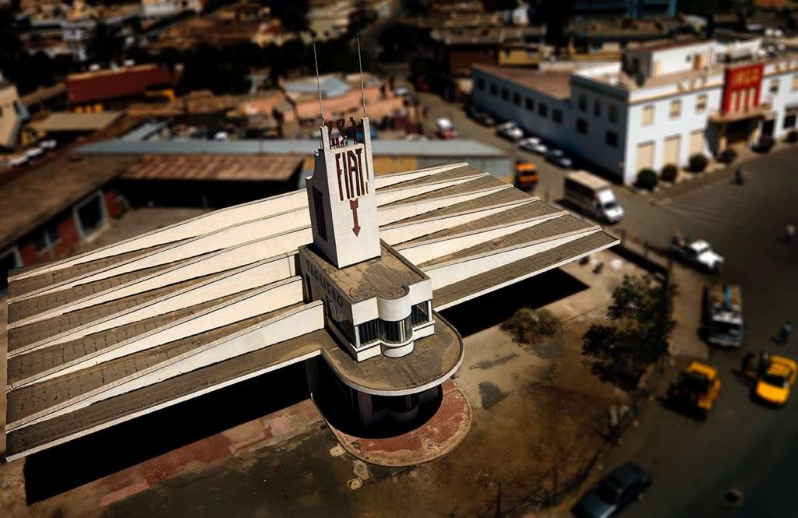
The airplane shaped Tagliero FIAT garage built by architect Giuseppe Pettazzi, in 1938, and similar to Frank Lloyd Wright's art. The building has 98 foot long concrete wings, stretching above the ground on each side of the pillars. For long time it was abandoned, but it may be turned into a bar soon.
